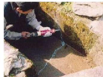
＜水路のひび割れ補修＞
