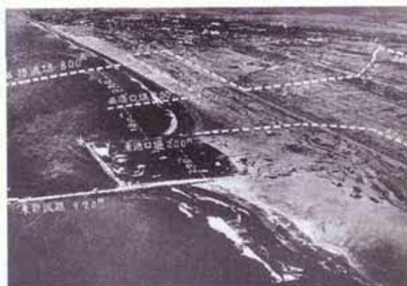
Fig. 6 Tomakomai port under construction(1955). (Ref. 3)
