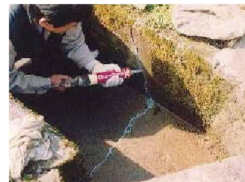
＜水路のひび割れ補修＞
