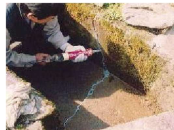
＜水路のひび割れ補修＞
