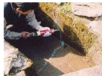
＜水路のひび割れ補修＞
